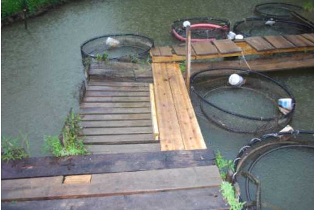
Figure 19. Rough, unfinished lumber nailed onto the surface of the dock made of weather-proof, treated lumber adds traction even when wet and helps to prevent slipping injuries.
