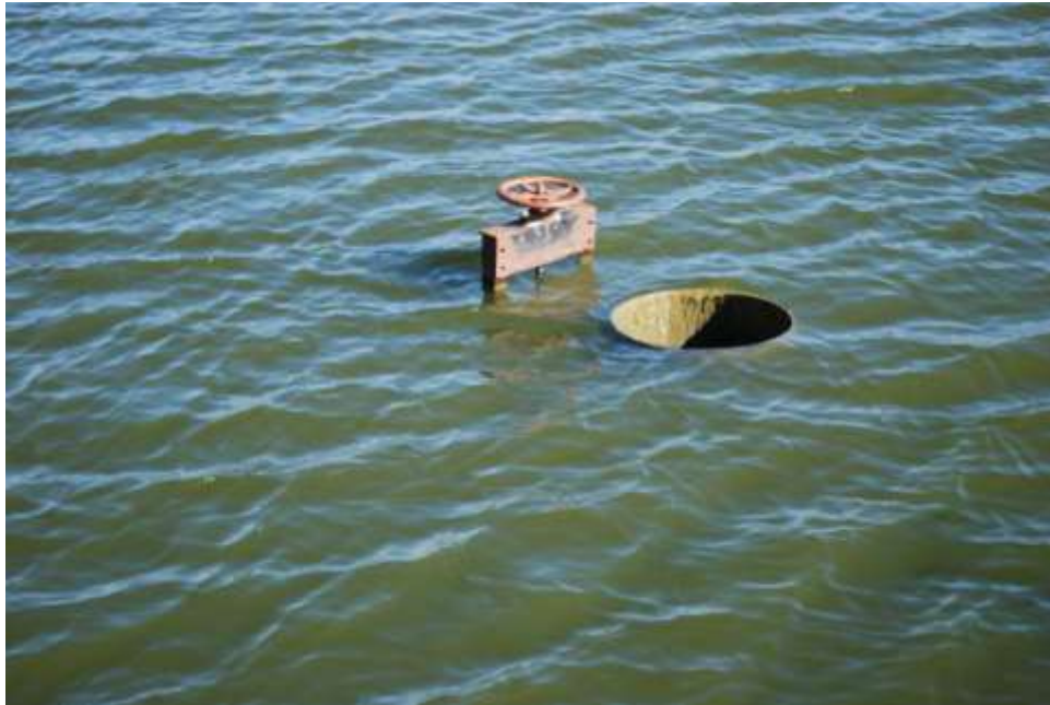
Figure 52. Water is drained or retained in this pond by raising or lowering a gate valve controlled by turning the wheel. In an incident in South Carolina during the past decade, a gate valve was inadvertently left open when the farmer was un-stopping a clogged large-diameter industrial pond drain. The stopped-up drain opening was underwater and was covered by a screen that had become overgrown with barnacles. To allow water to flow through the drain, the farmer cut through the clogged screen and was immediately sucked into the drain pipe and killed.
