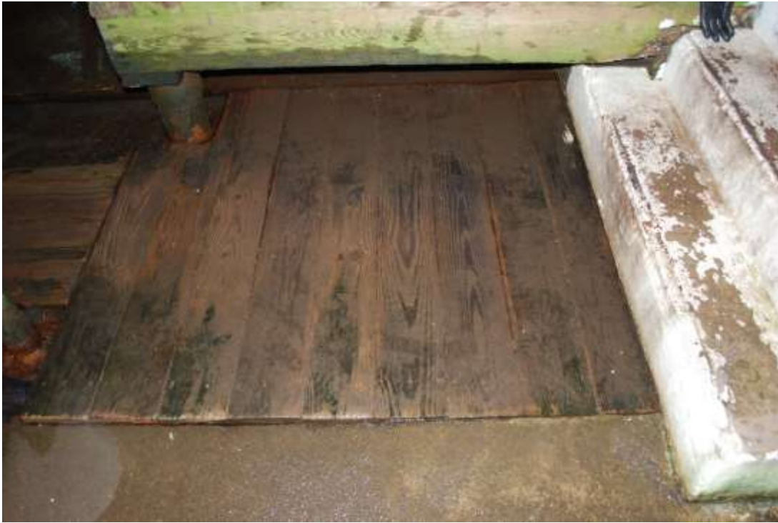
Figure 23. Wooden floors and walkways can be very slippery when wet and/or icy.
