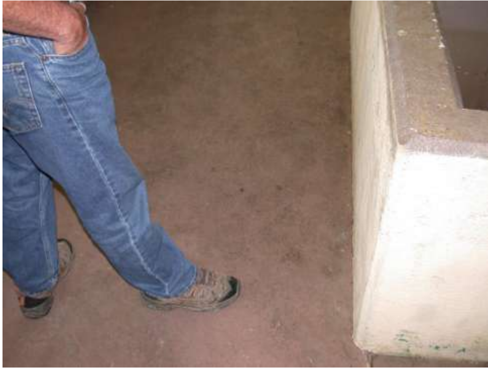
Figure 25. Wet floors in hatcheries can have better traction if grit/sand is put in the paint.
