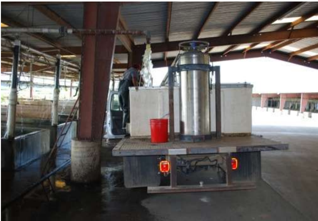
Figures 3 and 4. Water is pumped into tanks conveniently as the hauling truck drives underneath the water supply pipe. This alleviates the need for filling up tanks manually, bucket-by-bucket.
