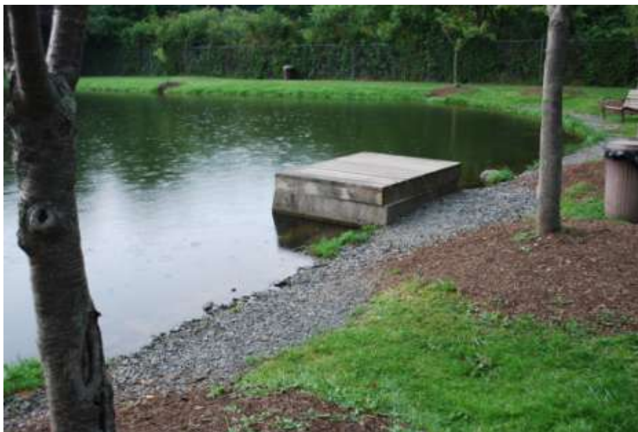
Figure 53. The pond drain at this pay lake is covered with a wooden structure to protect customers.
