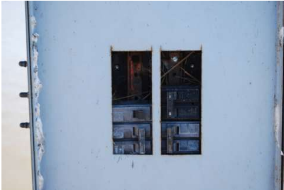
Figure 44. This electric fuse box cover is missing, and missing breaker switches expose underlying wiring.
