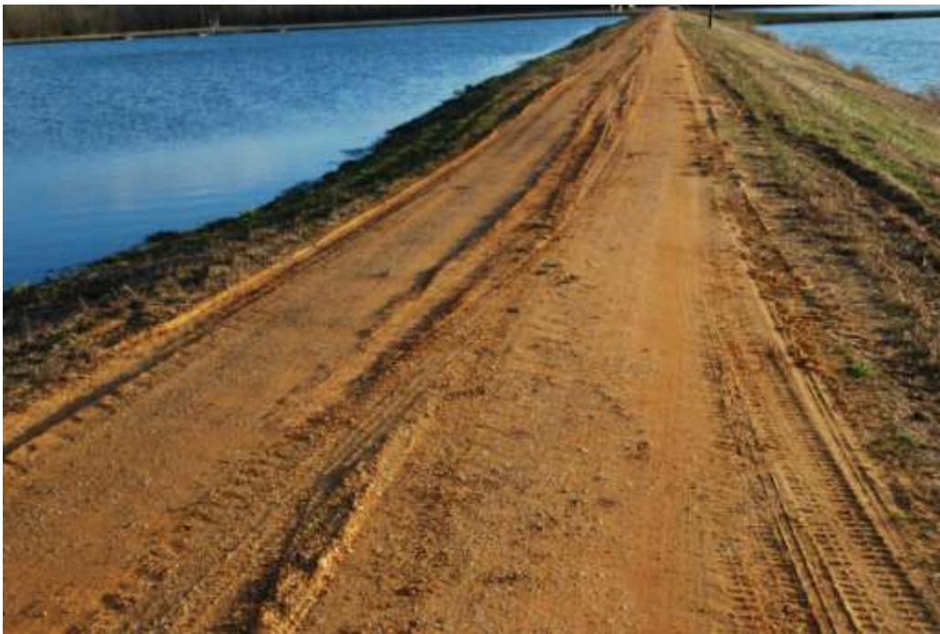
Figure 38. Gravel on levee roads reduces the chances of vehicles sliding off of levees or rolling over into ponds.
