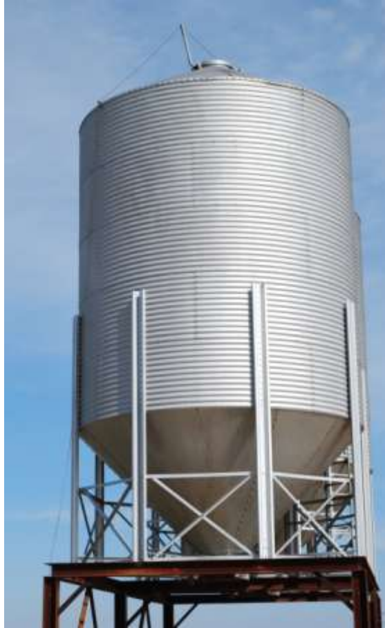
Figure 21. A chain attached to the hatch on top of this feed bin allows the bin to be opened for filling without having a worker climb to the top, minimizing the chance of a fall occurring.
