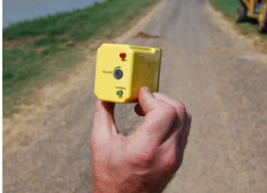
Figure 51. This ground fault interrupter (GFI, also called a ground fault circuit interrupter, GFCI) is used in the power box of a permanent electric paddlewheel aerator. On this farm, two workers were in the pond rewiring a paddlewheel aerator (all power was turned off while they were working on the wiring). After they finished the rewiring, a third worker turned the aerator on prematurely while they were still in the water (one waist-deep and the other ankle-deep). Both men received heavy electrical jolts, especially the worker who was waist-deep. The shock occurred because the workers had erroneously connected the ground wire to hot and the hot wire to the ground.
