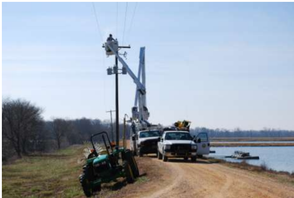
Figure 45. An electric company worker was holding power lines on an Alabama catfish farm when a co-worker unknowingly turned the power back on. It burned his right arm and half of his left arm; one complete and one partial amputation were needed. Workers could prevent this kind of incident by using a lock out – tag out system; the person working with the equipment that has electrocution potential locks the power switch in the off position with his own lock labeled by his tag. Only he can unlock this to turn the power back on after he completes his job.
