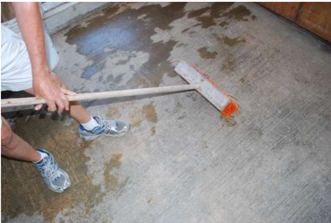
Figure 24. Rough concrete floors, providing traction even when wet, can be created with a coarse broom when the newly-poured drying concrete is still wet.
