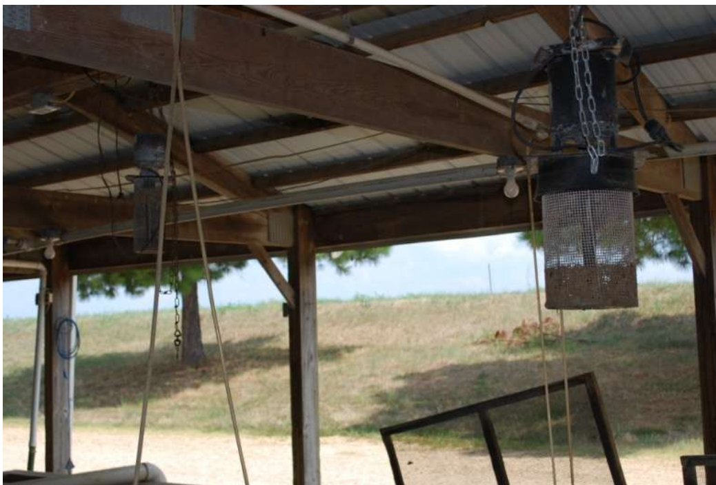
Figure 49. There is a greater risk of shock when electric-powered agitators are immersed in tank water. Many fish farmers report that they and their fish would frequently be shocked when they used these electric-powered agitators (“bull aerators”).
