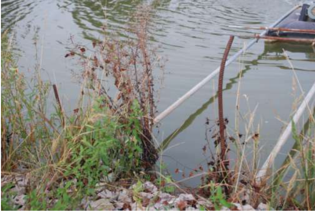
Figure 35. The tops of these rebar stakes used to secure the aerator are not capped or bent to protect against impaling.
