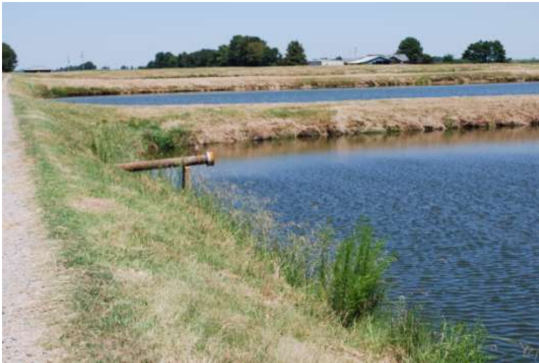
Figures 42 and 43. Levee erosion is more common around structures such as inflowing well pipes. Vehicles can drop off levees at eroded areas; adding to this problem, heavy vegetation growth hides the hazard (top photo). Mowing levees increases visibility, but steep levee banks (bottom photo) pose a roll-over risk (which can be decreased by using dual tires on tractors).
