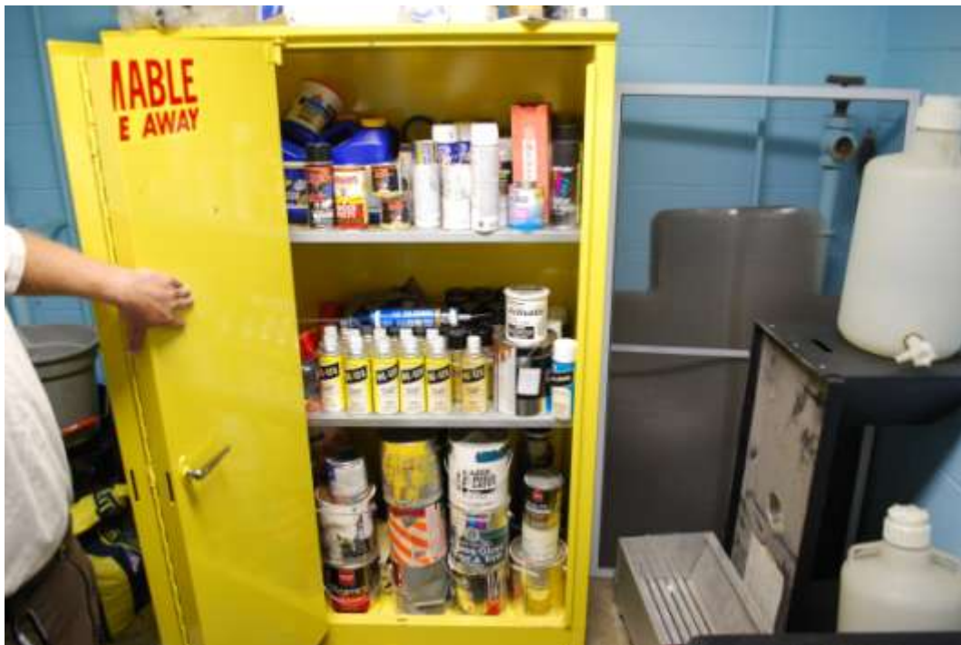
Figure 57. Flammable aerosols and paints should be stored in a metal cabinet.
