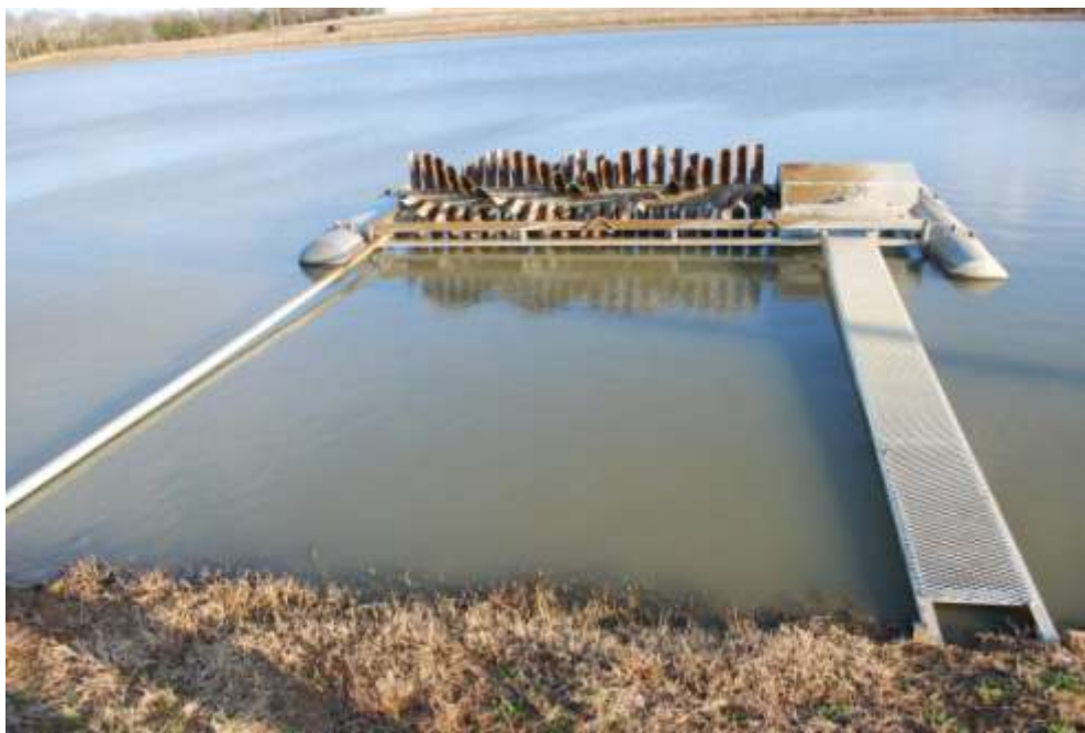
Figure 18. This metal "grip-strut" walkway to this floating paddlewheel aerator provides a safe way to access the electric motor. (Note: Although it is safer for workers to access and work on aerators using such a walkway, this also allows children to walk out to the aerator exposing them to potential injury.)
