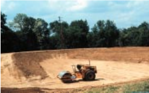
A new catfish pond under construction
